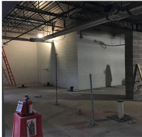
**Duct work hung in main mechanical room of academic wing. Copper piping completed in the art room, insulation to be completed next. Walls have been rubbed in the kitchen and block fill has commenced.**
