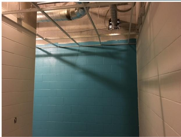
**Block fill complete in the gym. Chilled beams have been set in ceiling grid on lower level academic wing. Ceiling grid has been completed in the bathrooms of the lower level academic wing.**
