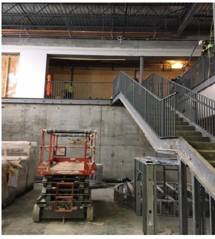
Casework installation is still progressing on lower level of the academic wing. The blue dry fall paint is completed in the cafeteria. Handrails are being installed in the library/maker space area. Also framing in library under stair stringer is complete as well.
