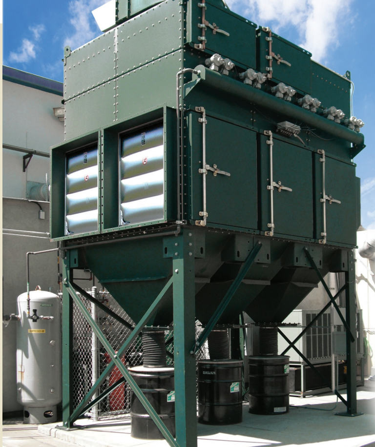
Left: Dust collector with explosion vent
